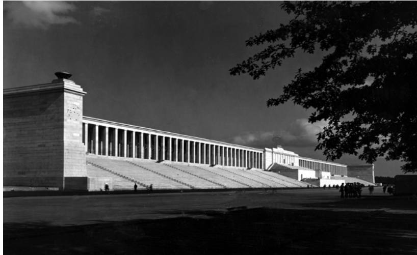
Fig. 1. Zeppelin Field Tribune – Nuremberg (designed by Albert Speer: 1935-1937); Stage façade [13].
